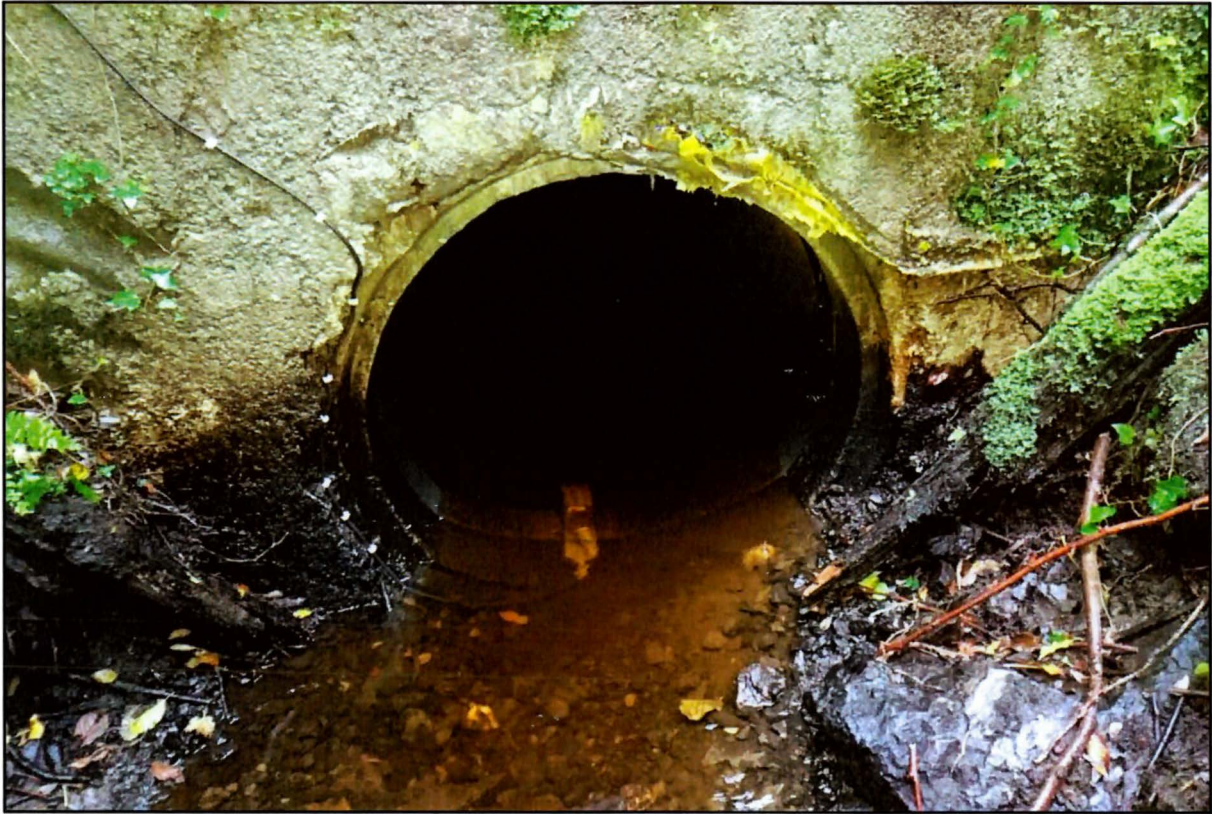
Photograph 3: Culvert 1 (downstream end) – Note Starflow flowmeter installed
